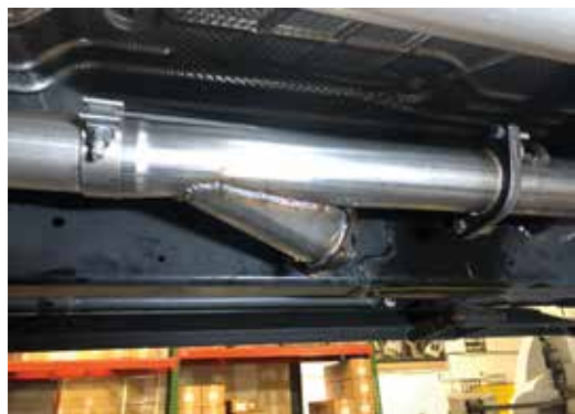
Image B: Aggressor Pipe Installed
