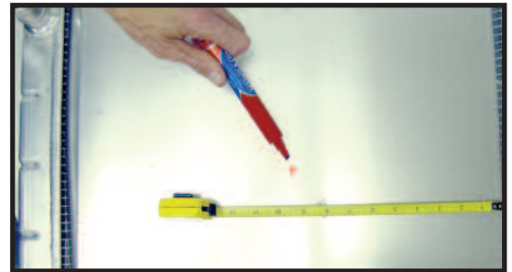
PHOTO 4: Mark fan center hub location.
